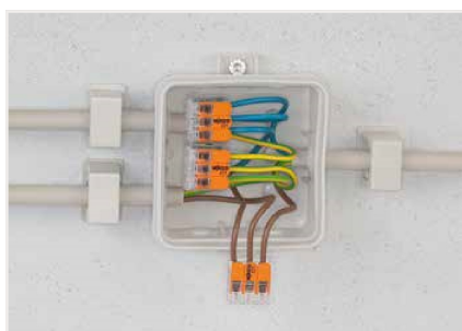
Wiring fine-stranded conductors in a junction box.
