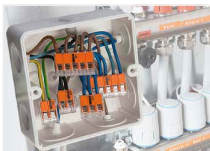
Wiring fine-stranded conductors in a junction box.
